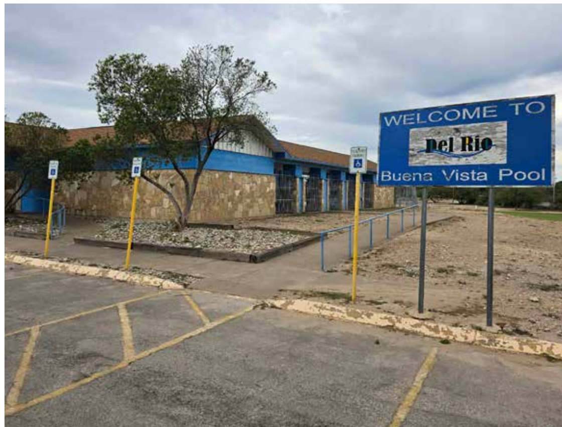
The Del Rio City Council is embroiled in conflict over the Buena Vista Pool project. (Photo by Joel Langton)
